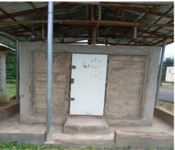
Figure 3: Evaporative cooling system
